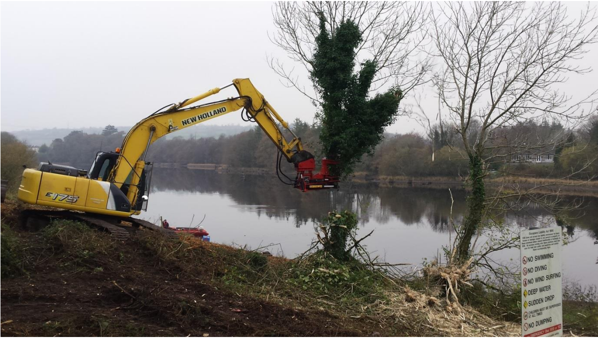
360 Excavator with tree shears attached at work
