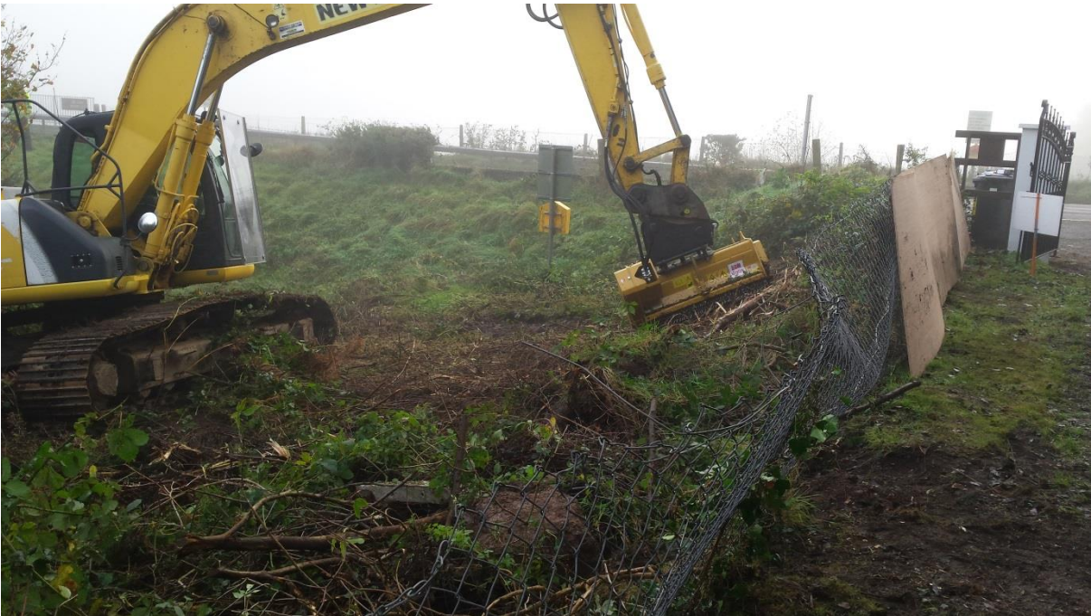
360 Excavator with Mulcher at work
