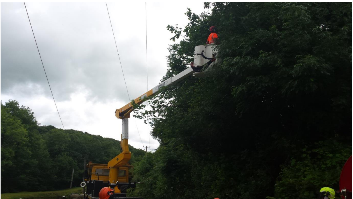
Hoist at work on Switch Out
